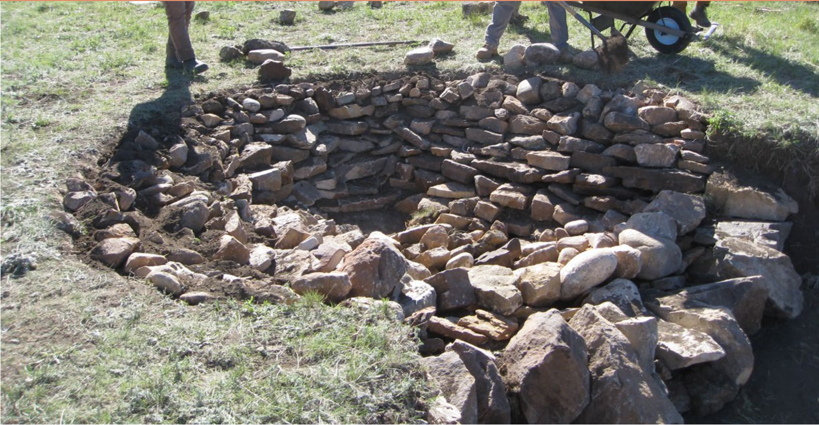
Zuni Bowl constructed by AWF at the Rio Mora National Wildlife Refuge in Watrous, NM. May 2019
