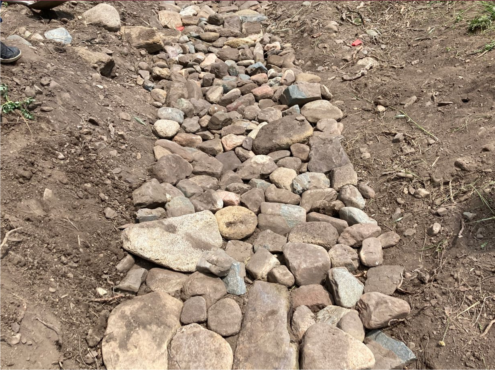
Rock Rundown constructed by HPWA seasonal crew in Sapello (Summer 2023).
