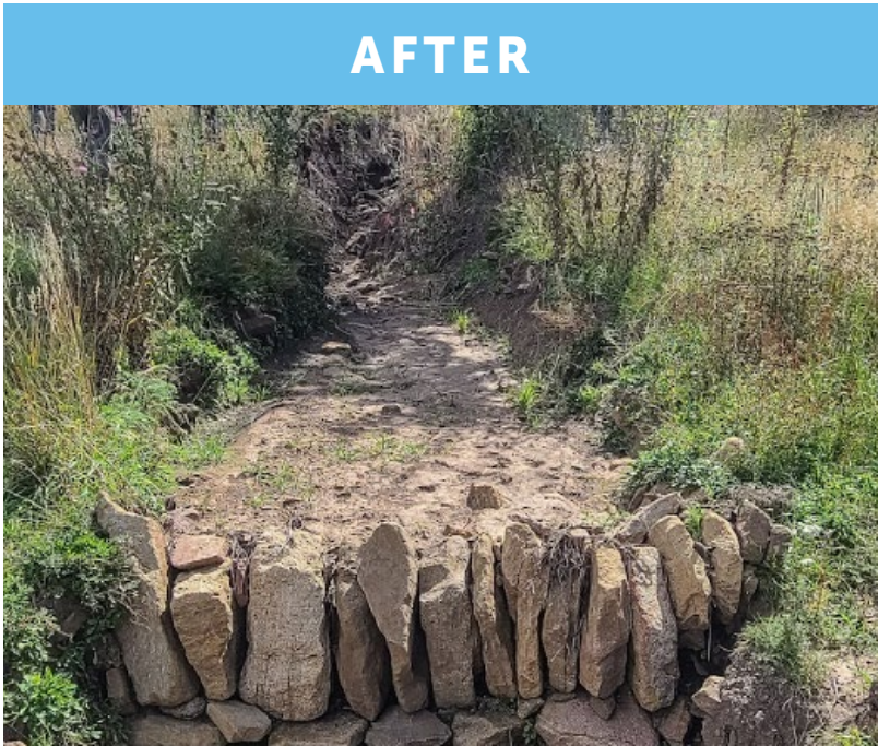
One Rock Dam constructed by HPWA seasonal crews in Sapello before (top) and after (bottom) filling up with sediment (Summer 2023).
