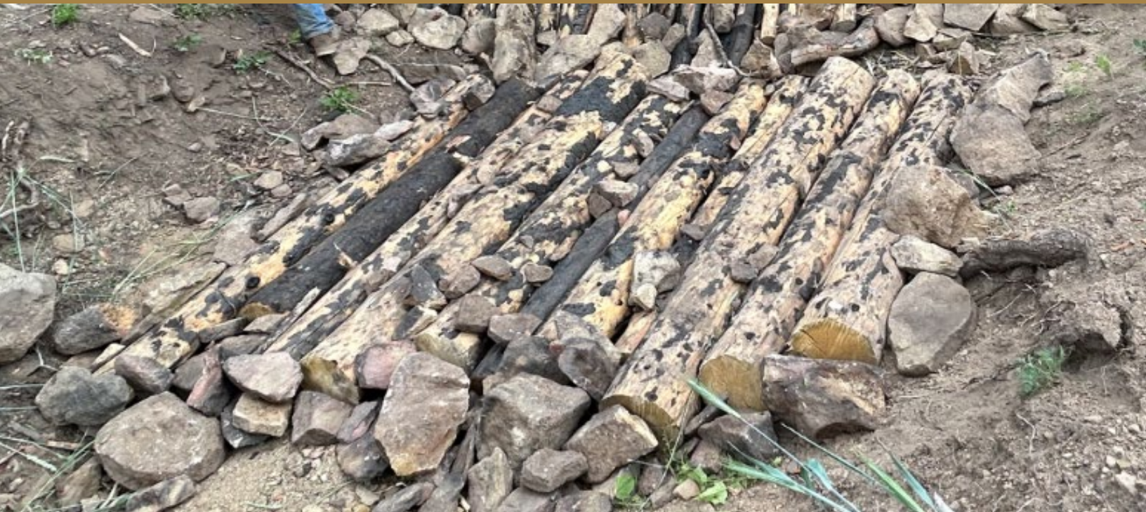
Log Mat constructed by HPWA and FSG seasonal crews in Sapello (Summer 2023).
