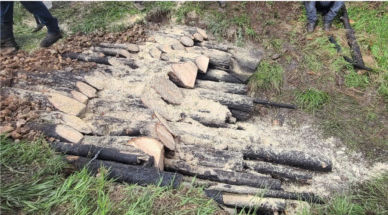
Log Step Down constructed by seasonal crews during training in Gallinas (Summer 2023).
