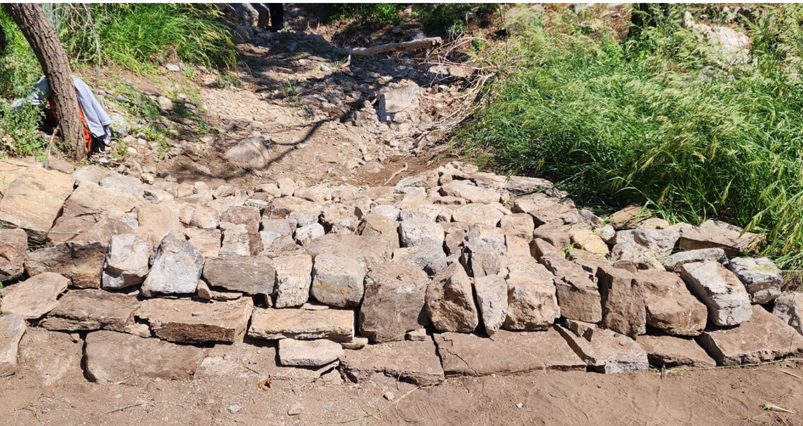
One Rock Dam constructed by HPWA seasonal crews in Gallinas (Summer 2023).
