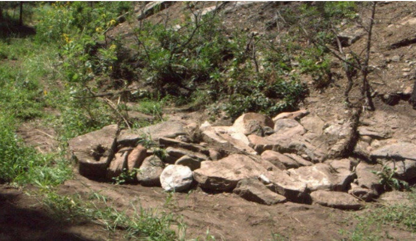
Baffle constructed by HPWA seasonal crews in Gallinas (Summer 2023).
