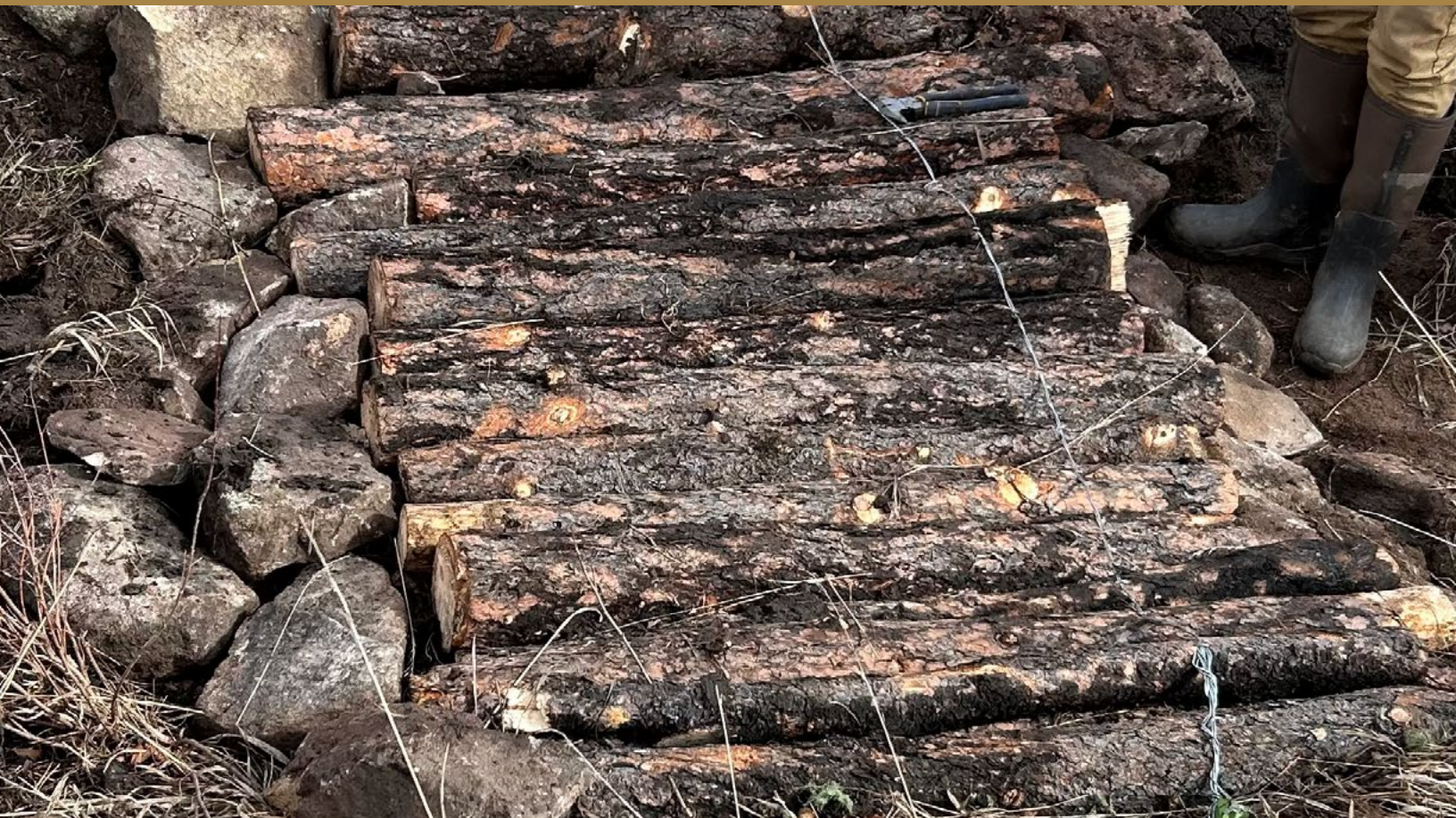
Log Mat to stabilize a channel side slope constructed by HPWA seasonal crews (Summer 2023).
