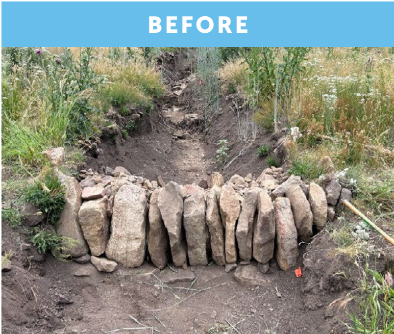
One Rock Dam constructed by HPWA seasonal crews in Sapello before (top) and after (bottom) filling up with sediment (Summer 2023).
