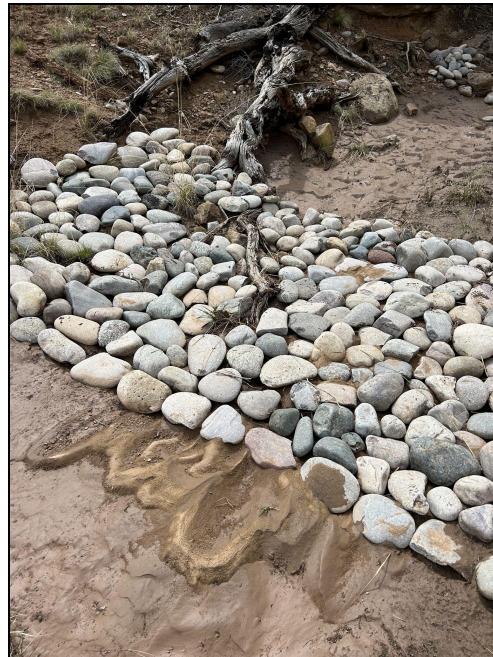
Figure 1: Rock rundown structure
