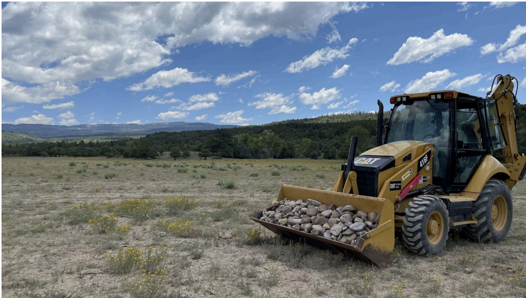
Figure 6: Backhoe transporting rocks to sites
