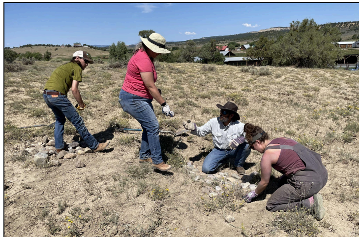
Figure 5: Participants learning how to construct rock rundown structures
