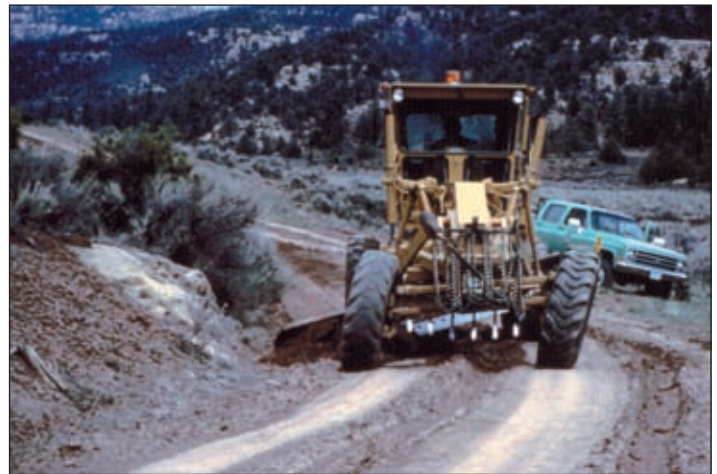
Photo V-3: Blading to maintain an insloped road template.
