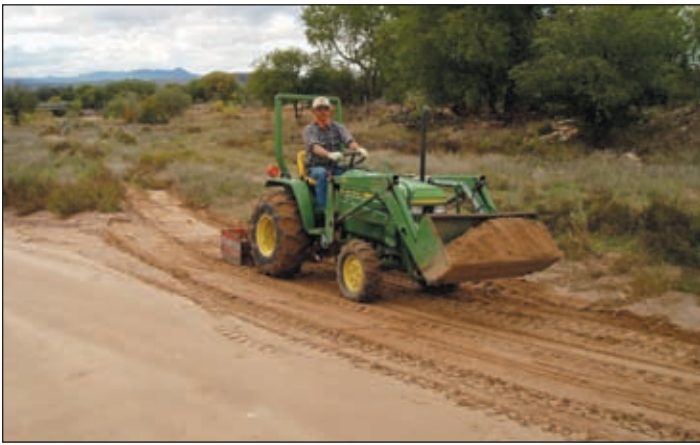
Photo IX-6: Farm tractor using a box scraper to make a lead-out ditch.
