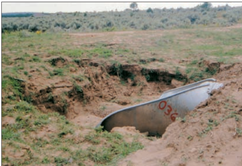
Photo VIII-2: Headcutting caused by improper culvert installation.
