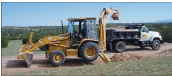
Photo IX-2: Backhoe removing sediment from a culvert inlet.
