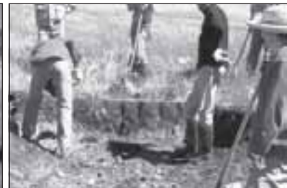
Installation of a log and fabric headcut structure on Holman creek meadow, September 2003
