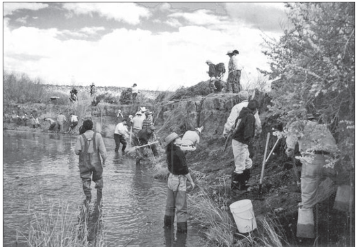
[Top] Riparian fencing to keep livestock out of the riparian zone. It has an electric top-wire to discourage elk from jumping in. The gates allow the livestock to use the area in the dormant season. [Bottom] Willow planting in April 2003. Three thousand willows were planted to stabilize the streambanks. (All photos with this article are courtesy of Jim Crosswhite, unless otherwise indicated.)
