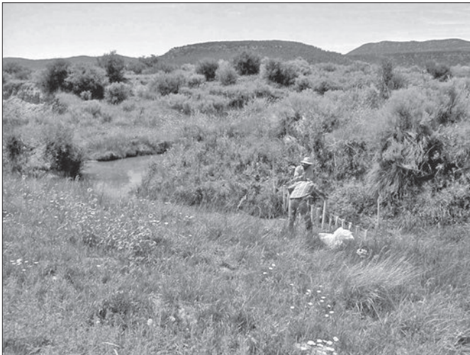
Post vanes designed by Bill Zeedyk were placed on Nutrioso Creek to divert water from eroding banks earlier this year.
