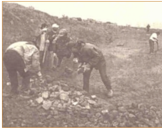
[Left] Members of RPMC join range users in covering the geoweb with soil. [Right] Rock is placed on top to “armor-plate” the area. (Photos on this page and page 9 courtesy of the BLM.)
