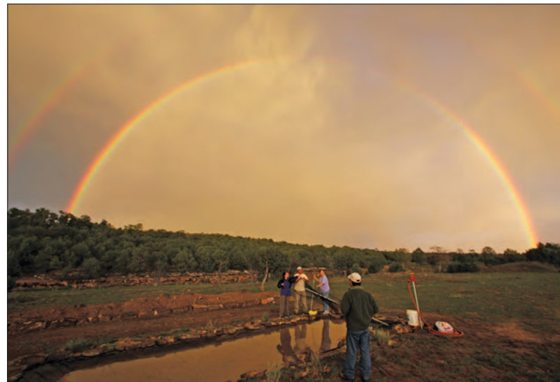
Placing bat netting over a completed pond, Valle Grande Grassbank, with double rainbow. © Courtney White
