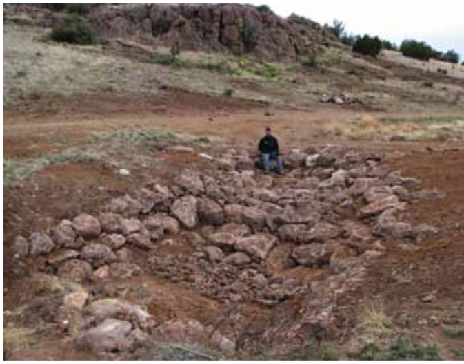
A “mega” Zuni bowl built by Craig Sponholtz to heal a headcut on Windmill Draw, Red Canyon Reserve, May 2010. (Photo by Avery C. Anderson)
