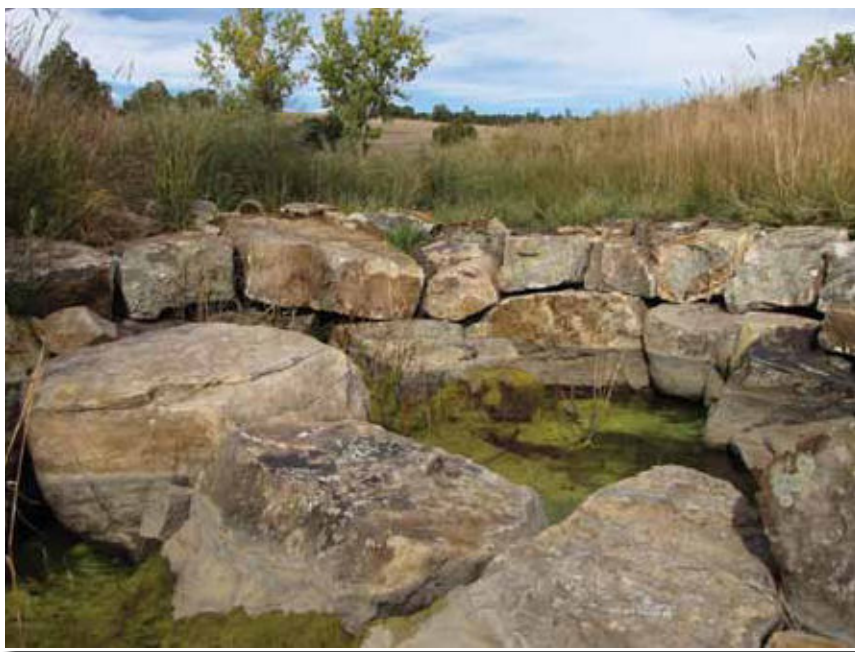
"The Frog Spa," Rock Lined Plunge Pool, Cañon Bonito Ranch, New Mexico, 2009. (Photo by Craig Sponholtz)
