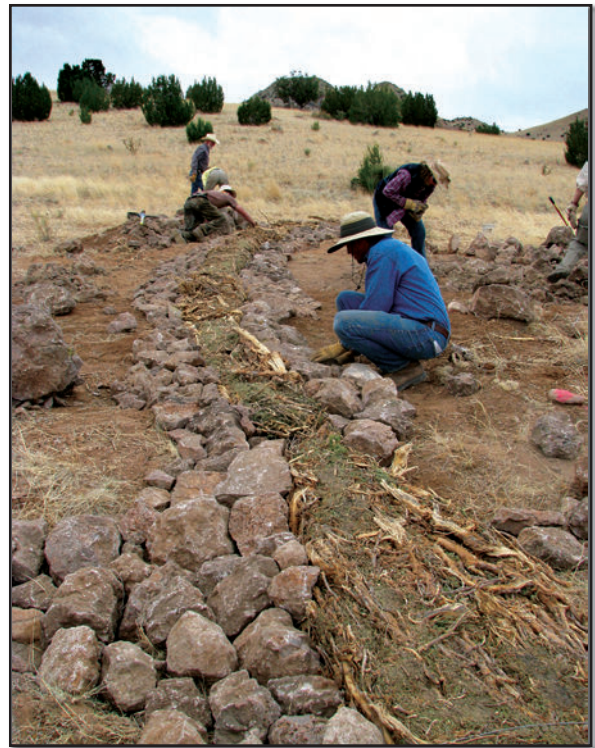
Upland erosion control structures installed May 2, 2009 by volunteers during a workshop on Red Canyon Reserve, N.M. Photo by Avery C. Anderson.
