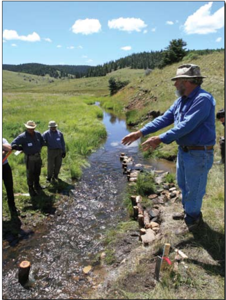
Bill Zeedyk discusses how a post vane protects an eroding bank on Comanche Creek in the Valle Vidal of Carson National Forest, July 2007. Photo by Courtney White.
