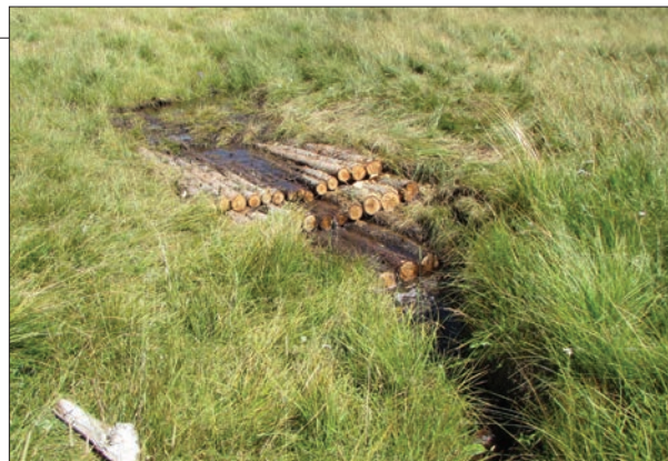
Figure 74. The log and fabric step falls schematic shows the detail of material placement (Zeedyk and Clothier, 2009). The log step fall in this photograph was built by volunteers in the Grassy Creek slope wetlands.
