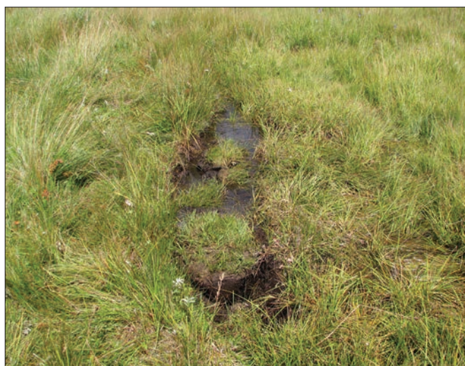
Figure 64. This sod plug, constructed by volunteers in the Grassy Creek slope wetlands, is slowing water flow in an incised channel cutting through the wetland. Water is spilling back over the wetland surface as seen in the photograph.
