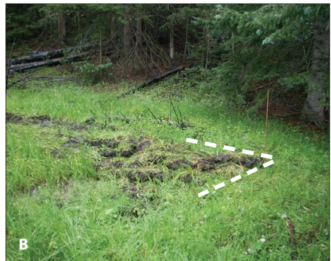
Figure 59 A. This photograph shows a log flow splitter leading to worm ditch in the Springwagon Creek drainage, Questa Ranger District, Carson National Forest, New Mexico, and was paid for by a 2011 River Ecosystem Restoration Initiative grant to the Quivira Coalition. Figure 59 B. This photograph shows a flow splitter constructed from sod. These may be used to spread water flow when the channel is not deeply incised.
