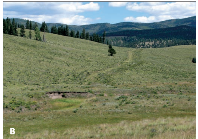
Figure 40 B. This photograph shows a road crossing a wetland complex in the Valle Vidal Unit of Carson National Forest, New Mexico (light green, lower left). Although the road has been closed and reclaimed, the damage it caused is still apparent as a large headcut where it crossed the valley floor. This is an example of a situation in which an initial stressor has been removed but the resulting degradation continues.
