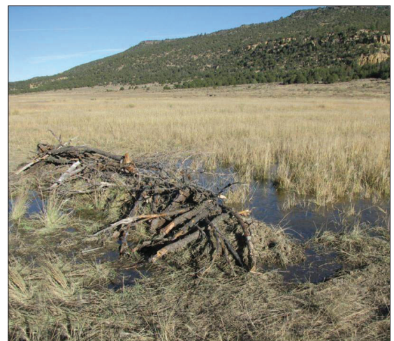
Figure 62. This burrito dam was constructed by volunteers at Cebolla Canyon near Grants, New Mexico.
