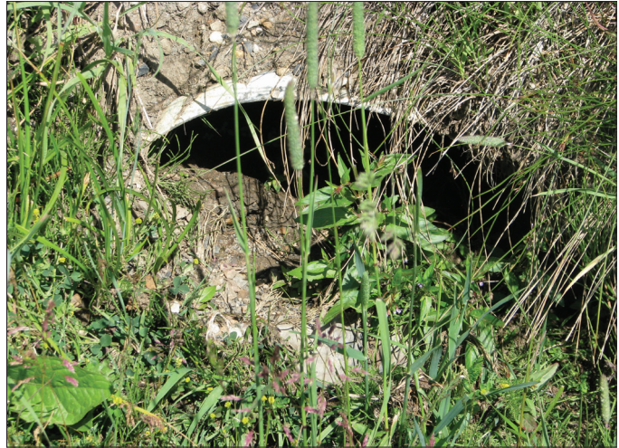
Figure 42. A blocked culvert will deprive downslope wetlands of water by diverting flow to another location.
