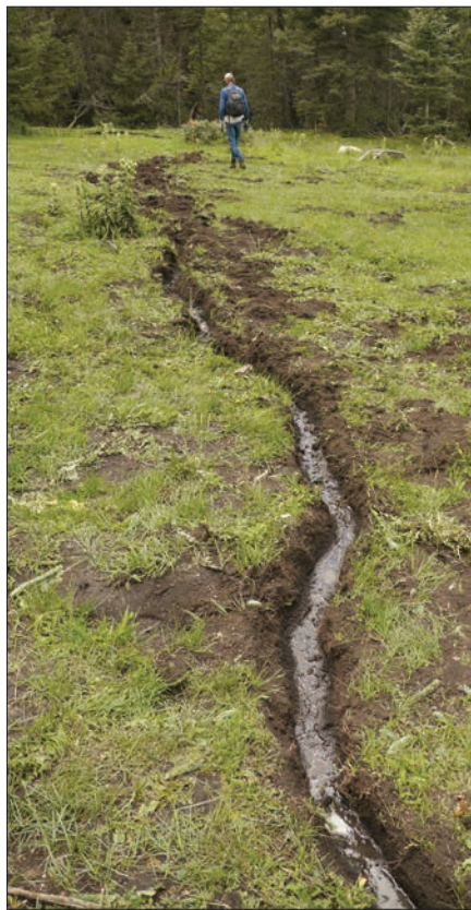
Figure 61. This lateral worm ditch was dug by volunteers in the Springwagon Creek slope wetlands in the Comanche Creek Watershed based upon design principles detailed in the schematic.
