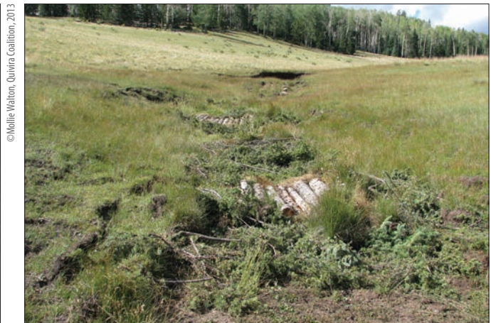
Figure 77. Log run downs may be used when the headcuts are shallow and in low energy systems. These log run downs are used to stabilize slope wetlands in the bottom of a gently sloping valley.
