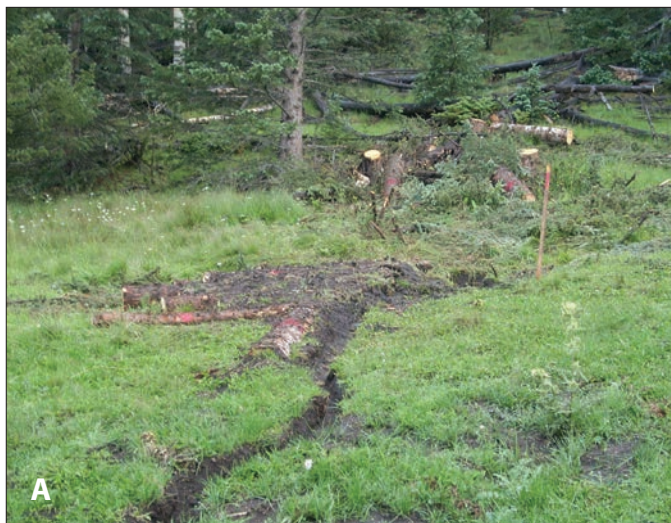
Figure 59 A. This photograph shows a log flow splitter leading to worm ditch in the Springwagon Creek drainage, Questa Ranger District, Carson National Forest, New Mexico, and was paid for by a 2011 River Ecosystem Restoration Initiative grant to the Quivira Coalition. Figure 59 B. This photograph shows a flow splitter constructed from sod. These may be used to spread water flow when the channel is not deeply incised.
