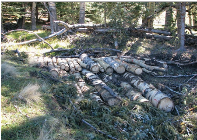
Figure 77. Log run downs may be used when the headcuts are shallow and in low energy systems. These log run downs are used to stabilize slope wetlands in the bottom of a gently sloping valley.
