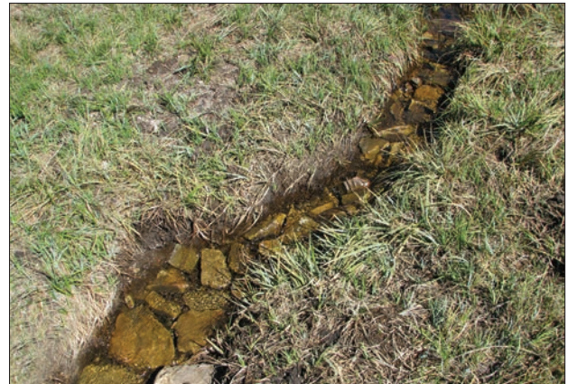
Figure 65. This channel liner raises the water level in a short reach of incised channel.
