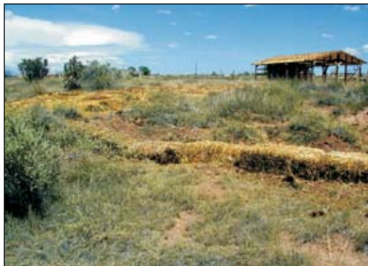
Strawbale headcut control on contour, Galisteo watershed, NM, 2001.
