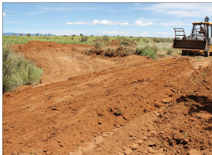
The first lift of the berm evenly spread.
