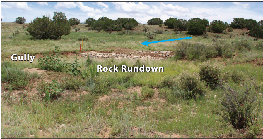
Figure 32. A rock rundown as a stable return site. Spreading stockpiled topsoil on the berm.
