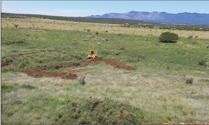
Initial stage of construction. Dozer is removing and stockpiling top soil from surface of borrow source .
