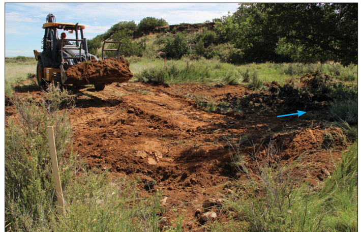
Backhoe hauling fill to start first lift of the plug . Stake at lower left marks the northwest corner of the plug .
