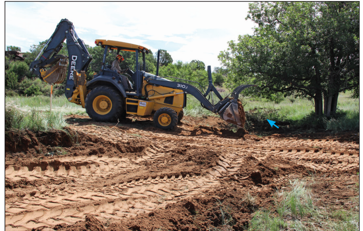
First lift upstream taper of plug in foreground has been compacted. Backhoe is adding fill to the downstream taper .
