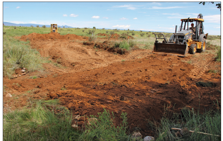
Final lift is spread. Note that the dozer in background is gathering fill from the surface of the borrow source for construction of the berm by the backhoe.
