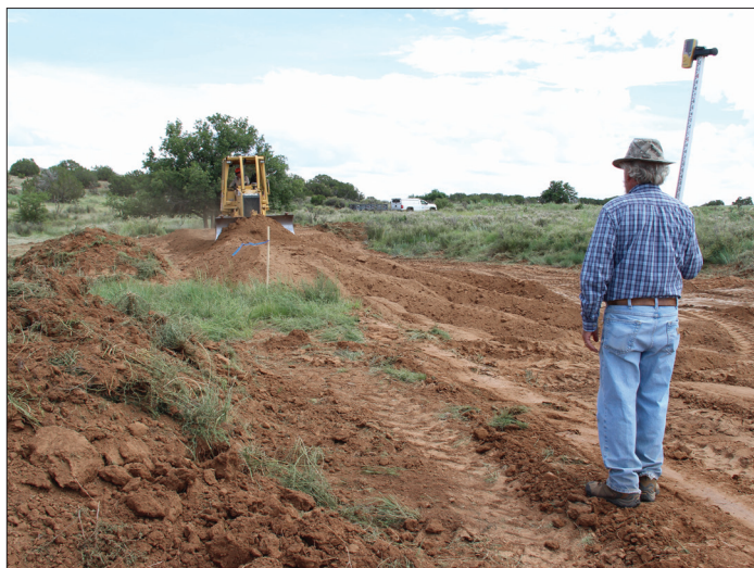
Checking elevation of berm against first cut at brim elevation.
