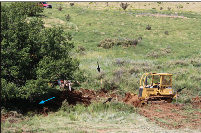
Dozer clearing topsoil from plug . Three of four stakes outlining dimensions of plug are visible in the photo.
