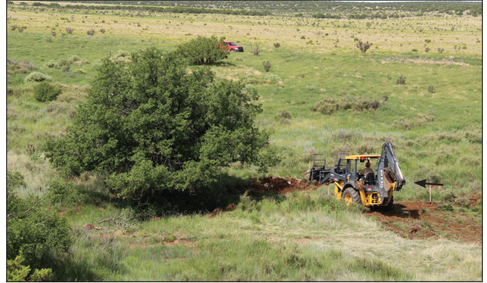
Backhoe removing brush from plug location. Lath stake marks north-east corner of plug .
