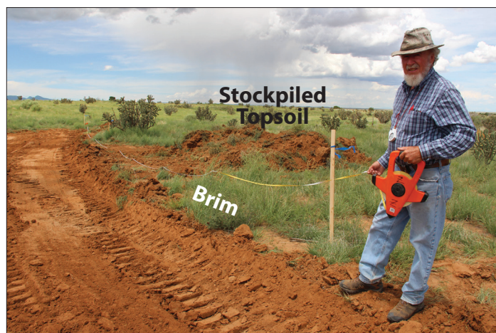
Measuring length of brim to check cross sectional area available to accommodate a flood event. Topsoil will be respread.
