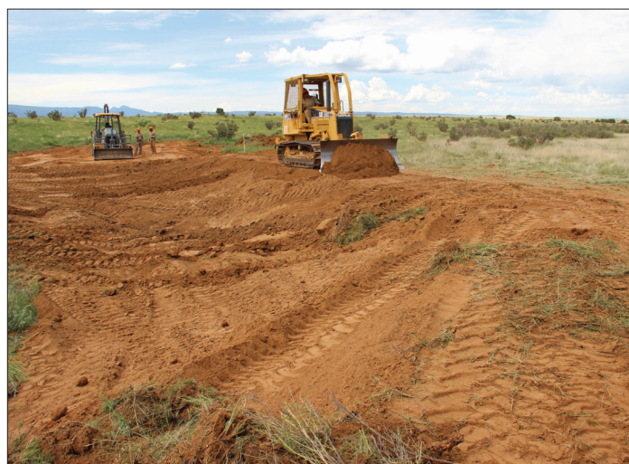
The berm nearing completion.
