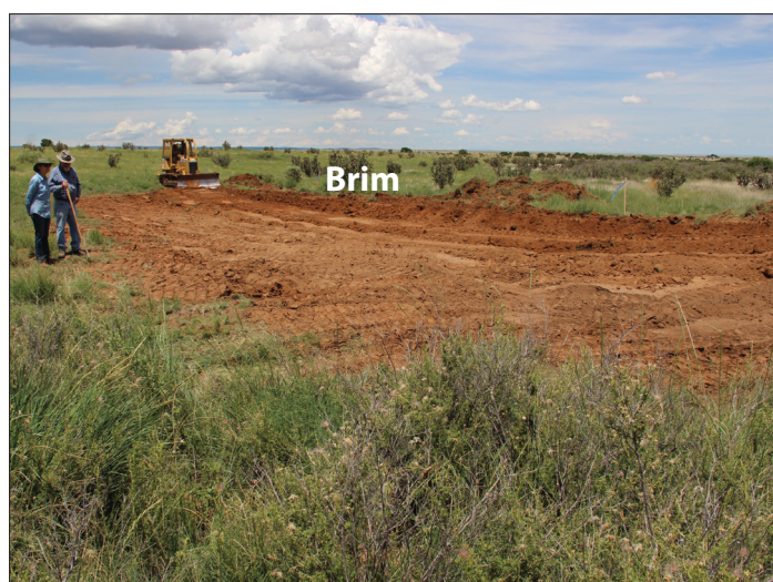
Dozer smoothing the surface of borrow source (bay) . Dozer located on valley left corner of the brim .
