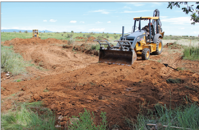
Spreading final lift, top of plug . Note that the top surface of the plug matches elevation of the top of the gully.
