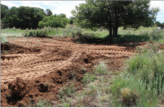
First lift of the plug completed and wheel-tracked for compaction of fill. Color of soil is due to a high clay content, which will pack well.
