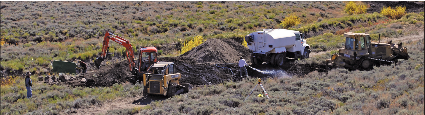
Equipment used on a project in Colorado includes a mini-excavator, skid steer, bulldozer and water truck. Water truck is being used to wet down fill material.
