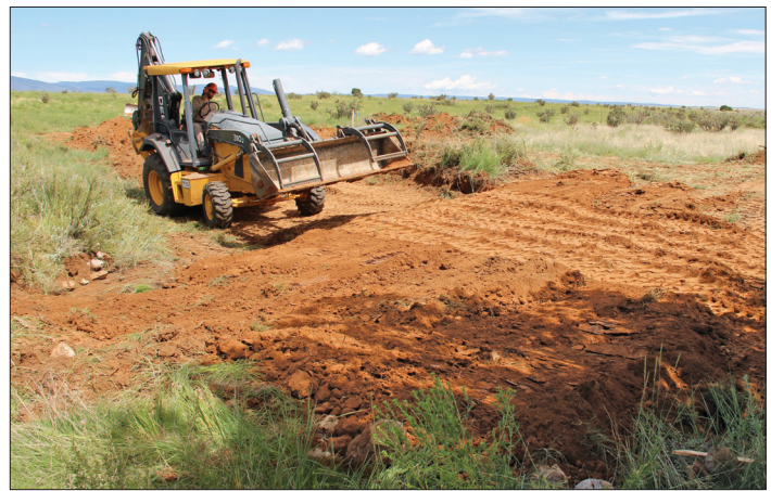
Tracking upstream taper and top of the plug for compaction. Note 3:1 slope on upstream taper .
