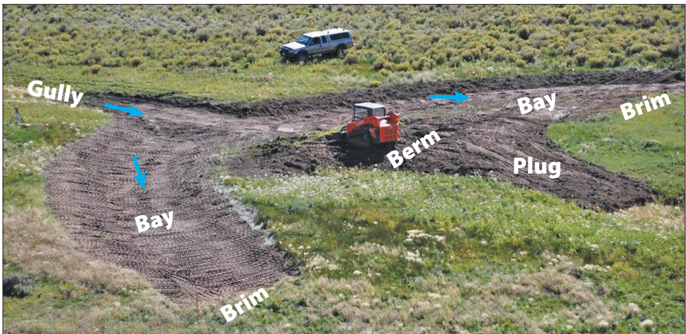
Figure 9. Key features of a typical Plug and Spread structure.
