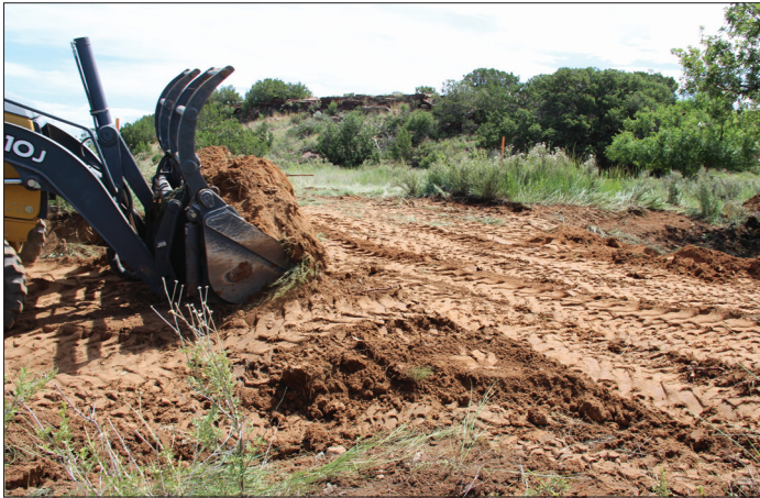
Adding fill to second lift of upstream taper .
