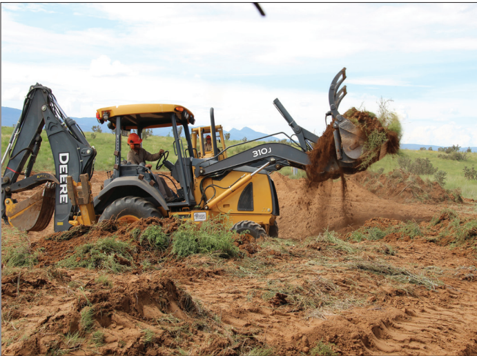
Spreading stockpiled topsoil back across finished surface of berm.
