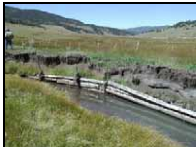
Figure 6. Revetment structure in Comanche Ccreek built in the late 1980s.
