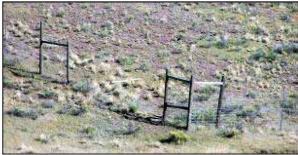
Figure 7. Pipe gate on large enclosure – this gate is too low to effectively exclude elk. Figure 8. South-east corner of fence is down allowing for cattle and elk access. Photos taken September 2005.
