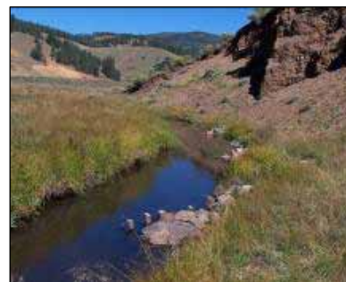
Figure 13. Three Vanes installed along an eroding bank during a 2004 work shop (Photo taken September 2005)
