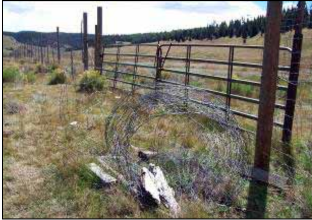
Figure 7. Pipe gate on large enclosure – this gate is too low to effectively exclude elk. Figure 8. South-east corner of fence is down allowing for cattle and elk access. Photos taken September 2005.
