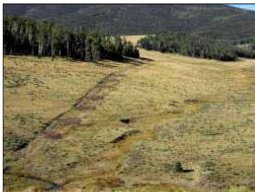
Figure 15. Rolling waterbars installed on an old road to the east of Gold Creek, September 2004.
