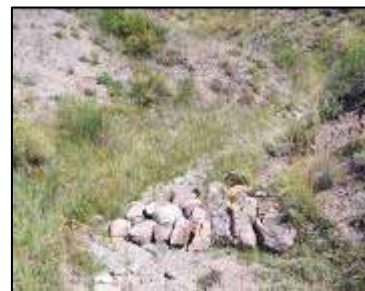
Figure 11. A Rock Baffle on Comanche Point Gully, installed September 2003.
