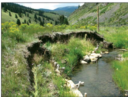
Figure 3. The same cut bank on Comanche Creek, after installation of post vanes.
